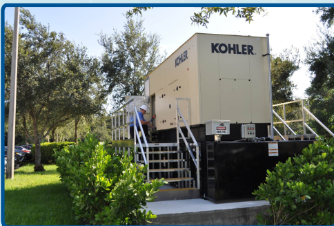
ALF Generator Installation- Palm Aire, FL
