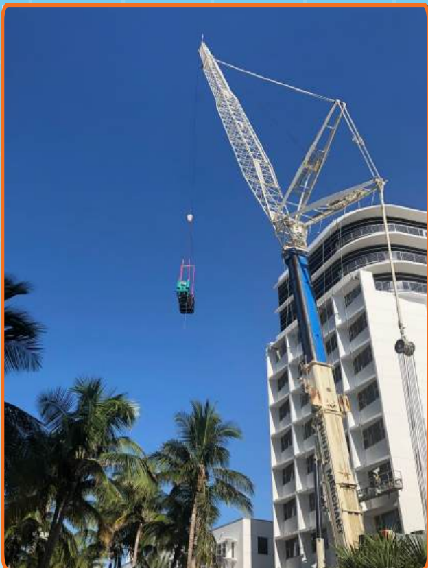
The Ritz Carlton 1500 KWGenerator Installation- South Beach, FL
