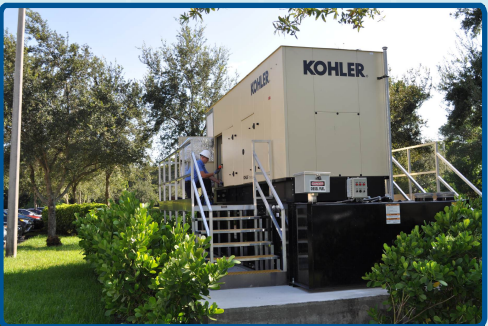
ALF Generator Installation- Palm Aire, FL
