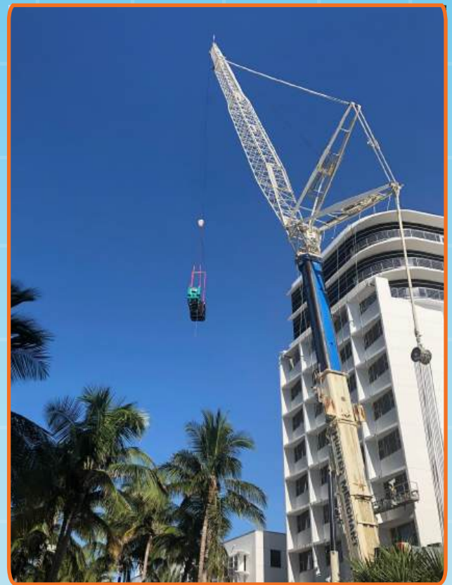
The Ritz Carlton 1500 KW Generator Installation- South Beach, FL
