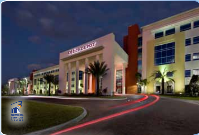
Office Depot World Headquarters Boca Raton, Florida- Complete Division 16 & 17 Electrical work 750,000 SF Building & 250,000 SF Parking Garage
