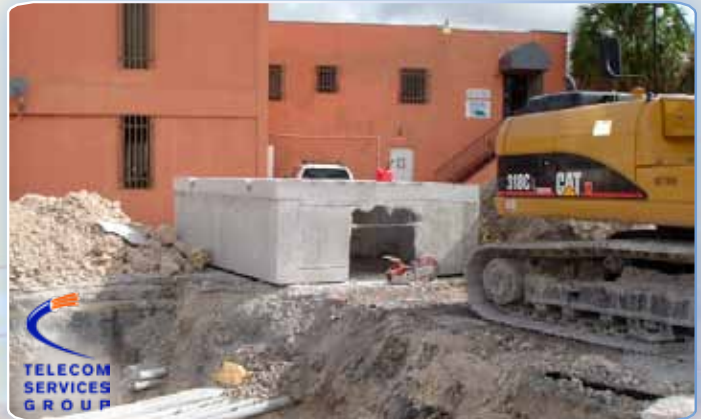
Miami River Bellsouth Telecom Miami, Florida
