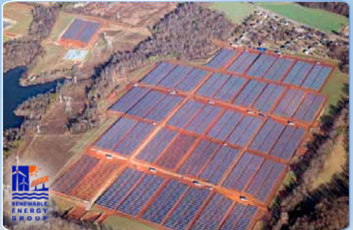
Utility Scale Solar Installation North Carolina 12Mw Solar Photovoltaic Ground Mounted Tracker System
