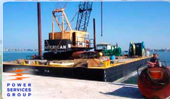
Robert's Bay Cable & Directional Bore Venice, FL Directional Bores, 1000 MCM Cable Placed
