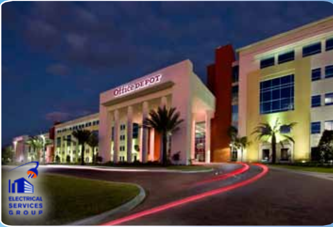
Office Depot World Headquarters Boca Raton, FL - Complete Division 16 & 17 Electrical work 750,000 SF Building & 250,000 SF Parking Garage
