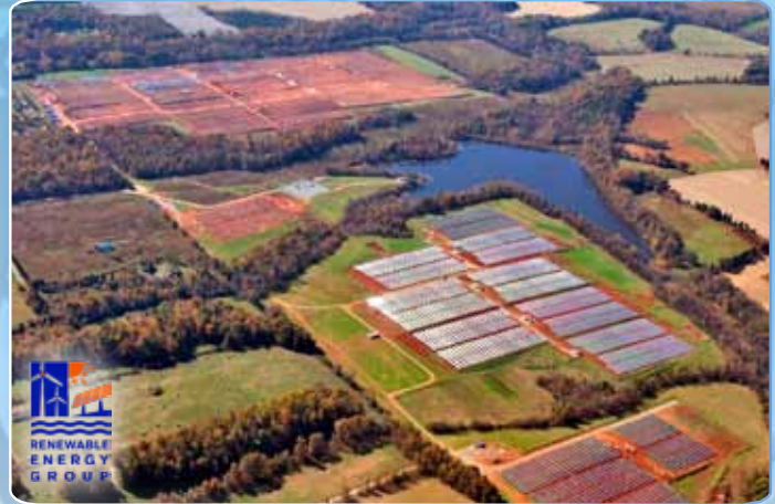
Utility Scale Solar Installation North Carolina 12Mw Solar Photovoltaic Ground Mounted Tracker System
